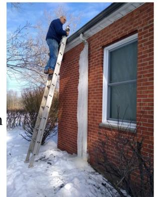
Roof gutters and drains were cleaned of debris before "real" winter arrived. The west side gutter of daycare did not get cleaned and was loaded with pine needles and cones. The triangle shaped screens made of plastic which keep debris from getting into the downspouts worked too well as the needles in the screens kept the water from flowing properly. We should consider taking the pine tree down to solve this problem. Currently we don't
